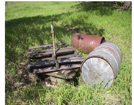
Poor wellhead protection and improper decommissioning can lead to contamination of a groundwater supply. Photo courtesy of SWA.
