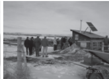
Barry Cocks, Empress, AB (403-565-2191) Solar/propane-powered winter stock water system from shallow well using shelter to house the water trough.
